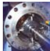
Hydraulikzylinder-Reparatur Hydraulic cylinders repairs
